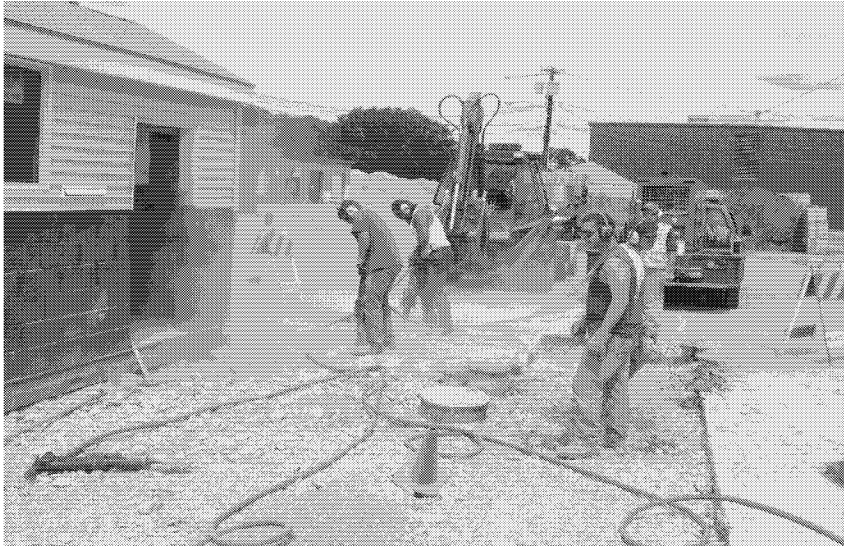
A new cement pad is installed at the Public Works yard
