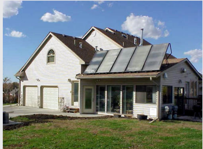
This residence in Missouri has five 4' X 8' solar panels installed. The panels, together with the solar green house, provide 40%-50% of the heating needs for the home during the winter and a year-round supply of domestic hot water. Photo: Ken Riead/NREL
